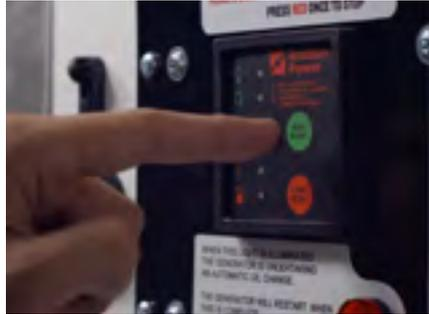
**2.** To start the generator, press the green button on the front of the cabin control panel once.
