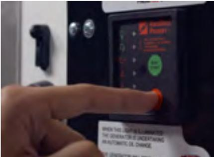
1. When you want to stop the generator, press the red button on the cabin control panel once.
