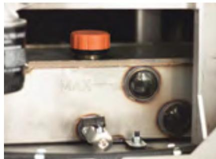
2. Check the oil using the two circular gauges found towards the base of the generator on the sump tank. The oil should be filled to the Maximum line marker next to the top gauge.
