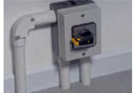
**3.** When the generator is running, set the Internal/External Power Switch to Position 2 for Internal (generator) power.
