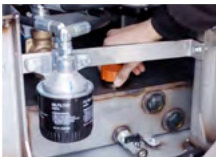
3. If your generator needs more oil, please remove the cap on top of the external sump oil reservoir that has the gauges on the front. Fill with suitable engine oil until the level reaches the maximum mark halfway up the top sight glass. Do NOT overfill. Always use the grade of oil specified in the appropriate RedBox generator manual.
