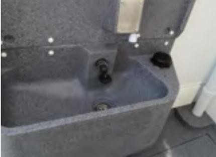
To fill the clean water reservoir in the hand wash basin, remove the filler plug adjacent to the bowl on the right hand side. Fill the reservoir with fresh clean water and replace the filler plug.
