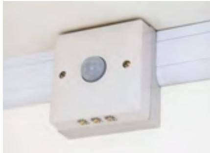
The toilet compartment contains a PIR operated ceiling light. The light will operate when a person enters the toilet room, and will turn off when the person leaves the compartment.
