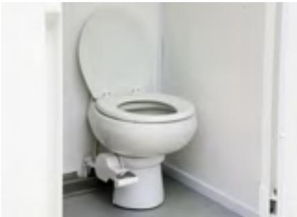
Your cabin is equipped with a toilet with fresh water micro flush. To operate the toilet flush, raise the flush lever to add water to the toilet before use, then after use hold down the flush lever until the contents leave the toilet. Allow the flush lever to snap back which permits positive sealing around the flush ball. A small amount of water should remain in the bowl.
