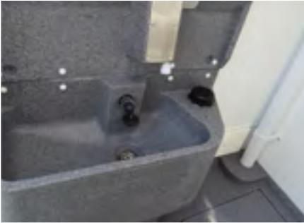
The hand wash basin in the toilet has its own clean water reservoir held within the base pillar. See 7A.8 for advice on filling and emptying.
