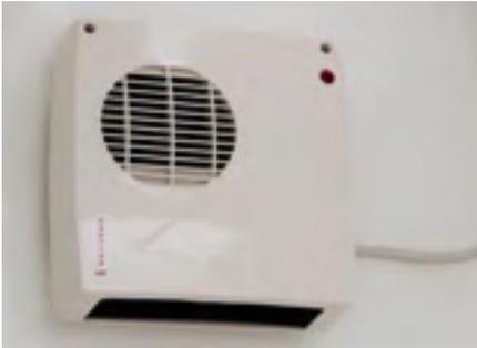
The toilet compartment is equipped with a fan heater. To operate turn on the wall mounted Fan Heater isolator switch. Pull the cord to switch on or off. The unit is not thermostatically controlled.
