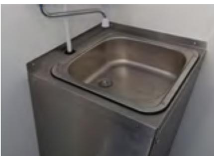
Units with fresh water toilets are fitted with stainless steel sink basins. The water for the hand wash basin is pumped automatically from the clean water reservoir to the instant hot water unit. If there is no water in the clean water tank, the pump will not operate. See 7B.7 for how to check and fill the tank.
