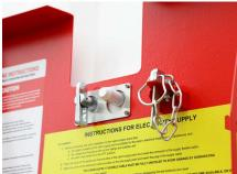
1. Release the anti-loose fastener and safety pin.
