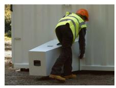
**3.** Once in position, lock the cover. Remove the keys and close the lock seal to protect against dirt or damage.
