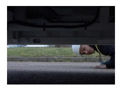
1. Make sure your cabin is situated on firm level ground able to support the weight of the unit. Inspect the ground underneath the unit and check there are no items which may damage the underside of the unit.
